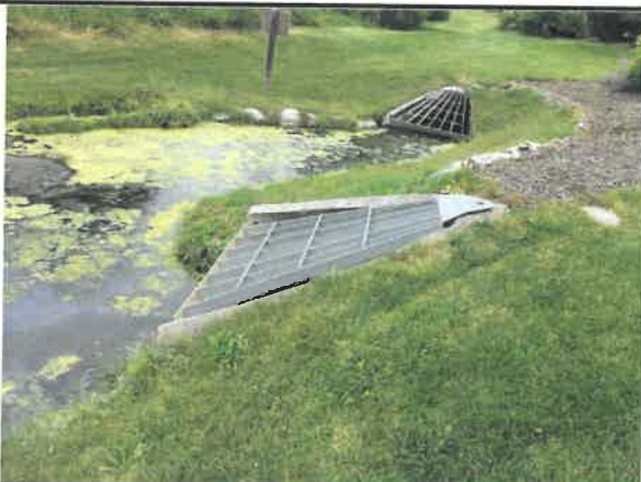
Side view of outfall structure
