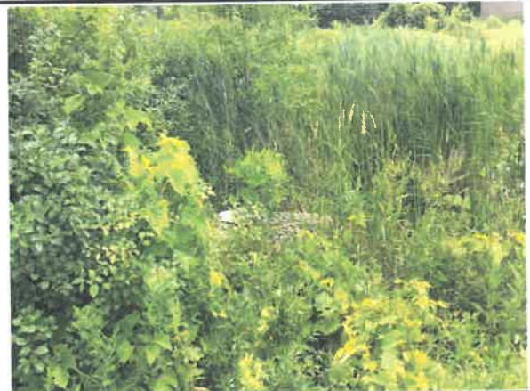
Side view of outfall structure
