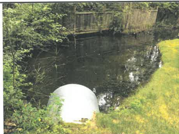
Easterly view of outfall structure looking westerly at release side of structure
