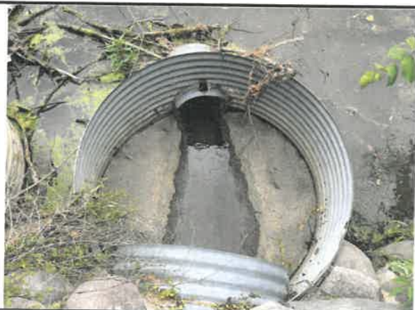
View looking down onto outfall
