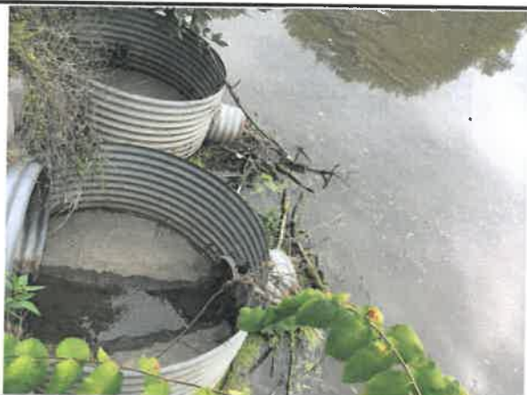
Southwesterly side of outfall looking northeastern
