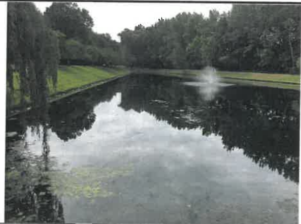
Northeastern side of basin looking south
