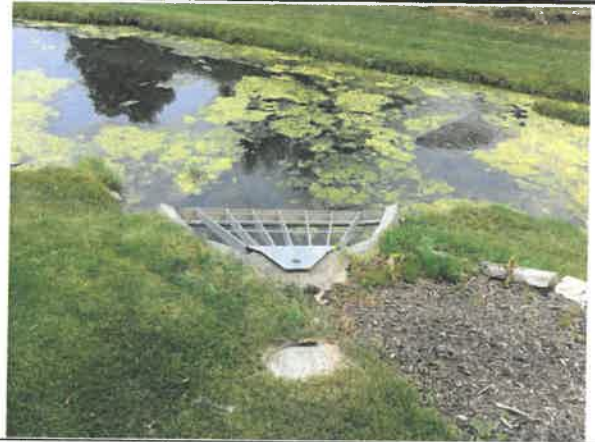
Top view of outfall structure
