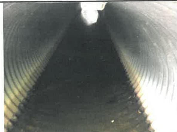
View into structure
