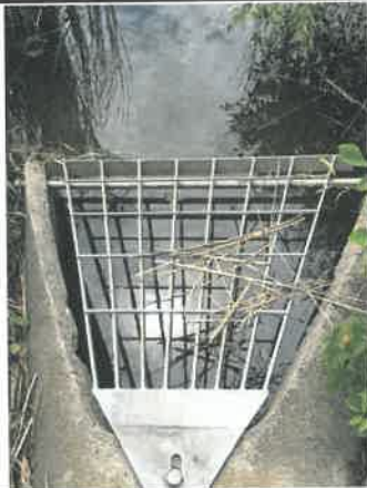
Top view of outfall structure
