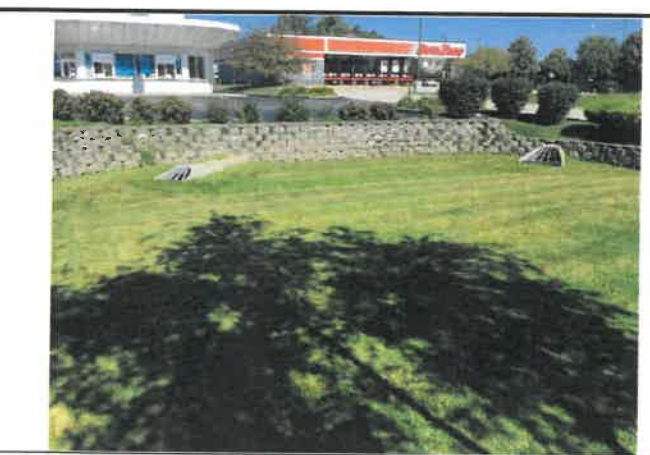
Southeasterly side of basin looking northwesterly
