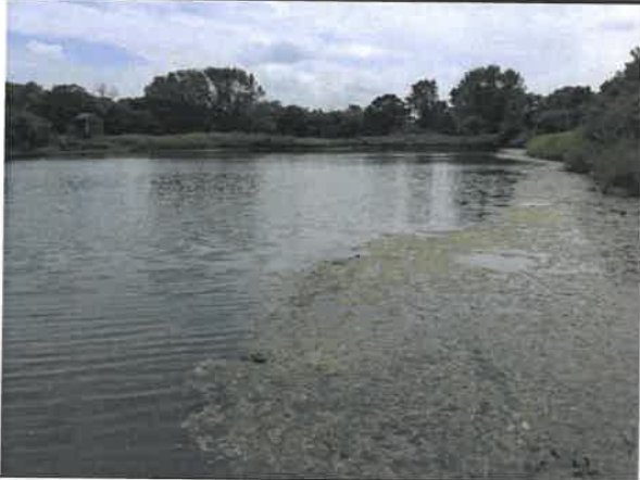
Northeastern side of basin looking south
