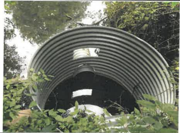
View into outfall structure
