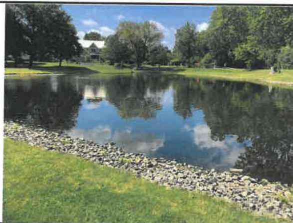
Easterly side of basin looking southerly
