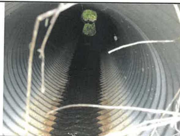
View into outfall
