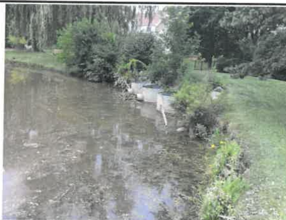
Northeastern side of outfall looking southwesterly
