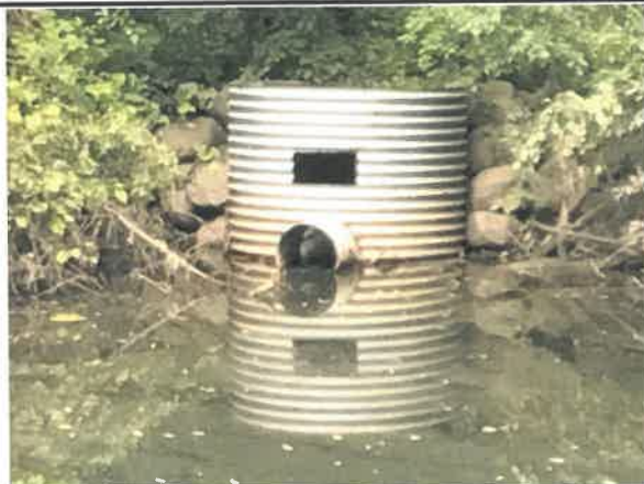
Easterly view of outfall structure looking westerly
