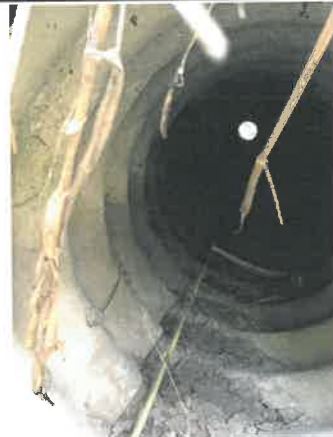
View into outfall structure
