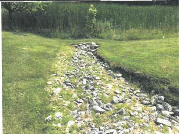
Southerly view of trench
