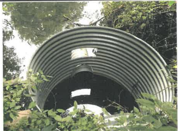
View into outfall structure
