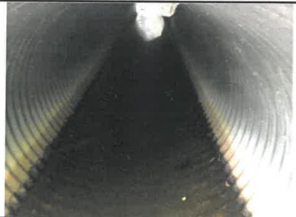
View into structure
