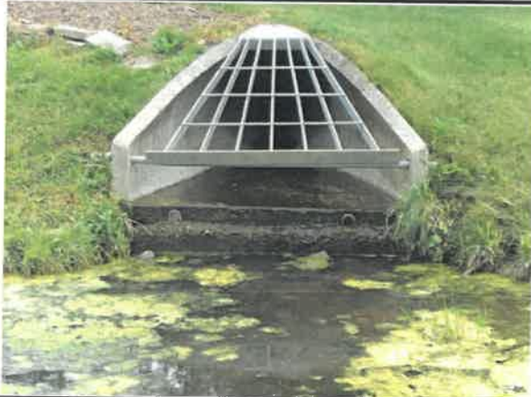
View looking into outfall structure
