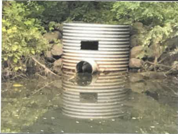
Easterly view of outfall structure looking westerly
